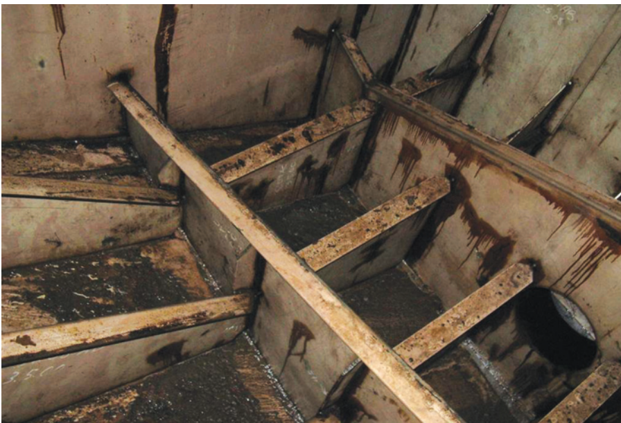
Image 1: The forward day tank of a Lloyds + 100A1 Class Tug undergoing cleaning due to bio-mass contamination.
